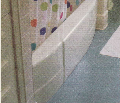
The Wears will cover the ASBESTOS TILE with natural linoleum and keep the existing ceramic wall tiles.
